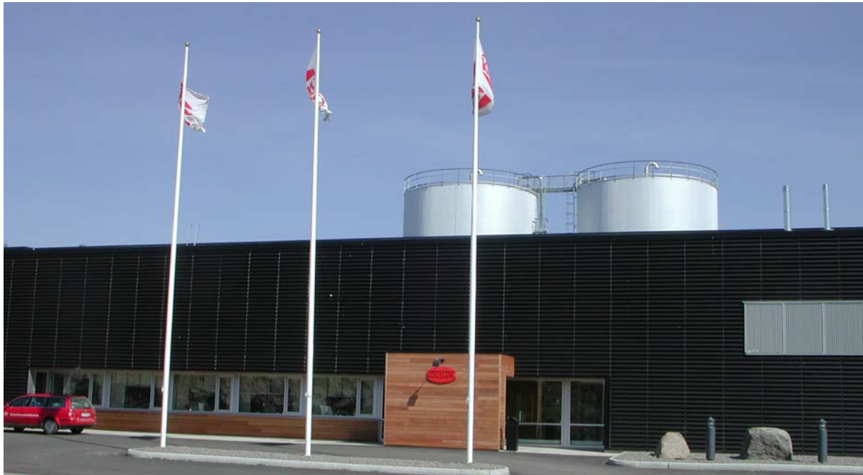
The entrance of the Biomal plant.
